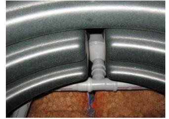
**Check that the water distribution pipe provides an equal distribution of water to the BIOROCK media***To be done annually*
